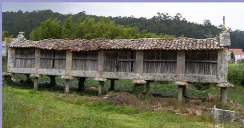
**An architectural design for drying and storage of maize using renewable energy: the hórreo**
